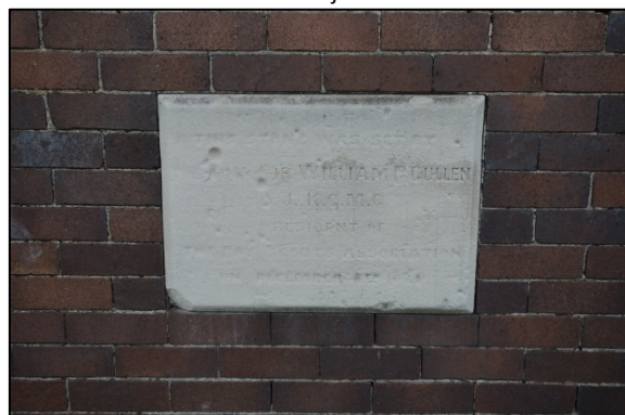
Figure 18. Foundation stone. Note that the text is significantly eroded.
