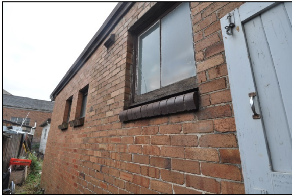
Figure 21. View of western façade. Note the c1970s extension evident from variation in brickwork and simplified window sills.
