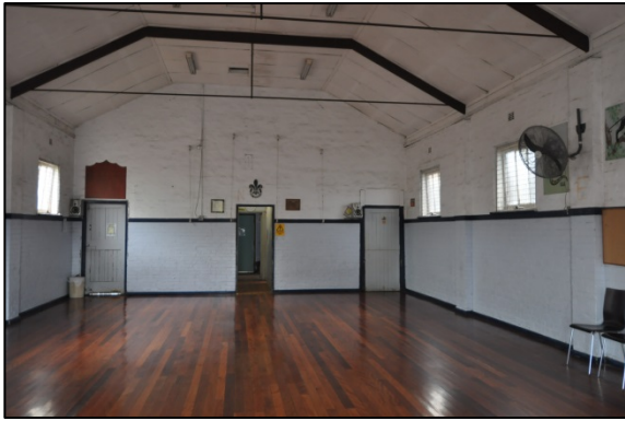
Figure 24. Interior view of original Scout Hall building.
