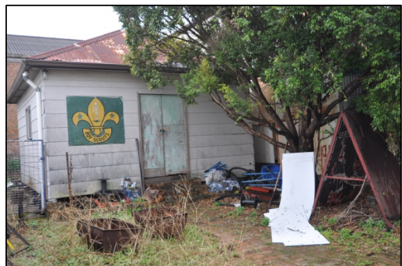
Figure 31. View of outbuilding. Note that Rappoport did not gain access to the interior.
