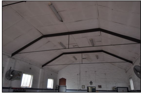
Figure 25. View of ceiling showing fibro panels, truss.
