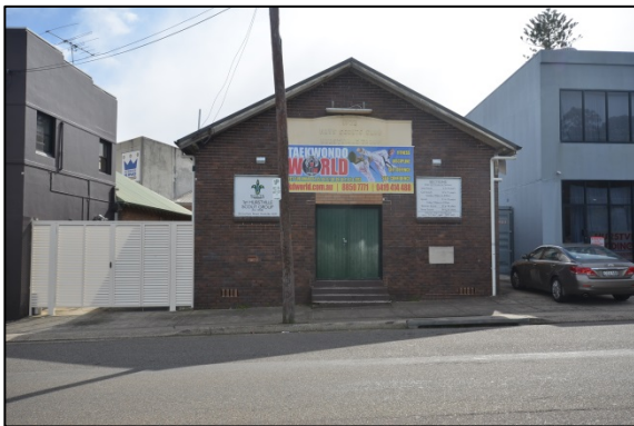
Figure 15. View of the subject site.
